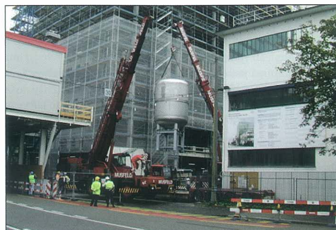
Placing a vessel in the pit under the future main entrance.
