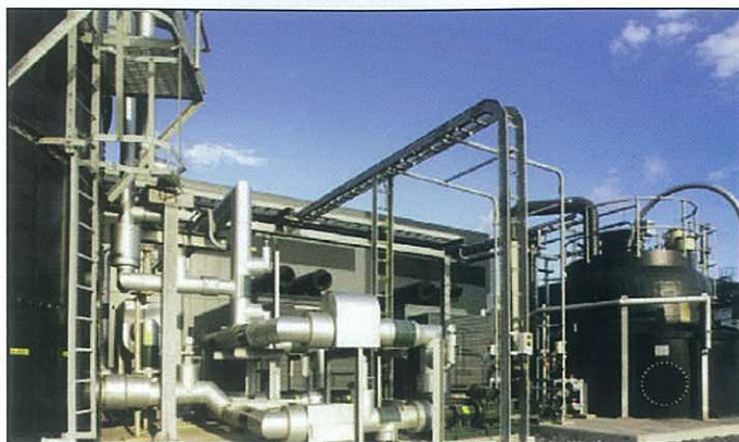
Centocor Biologics Ireland: Facility to capture rainwater from roofs within a grey water recovery system for future use in sanitary and ancillary process applications.
