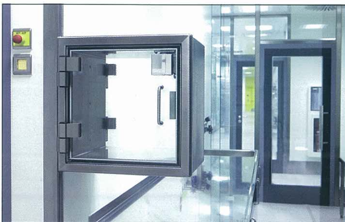
Material locks in the wall ensure short ways for the transfer of samples and documentation to the analytical department.
