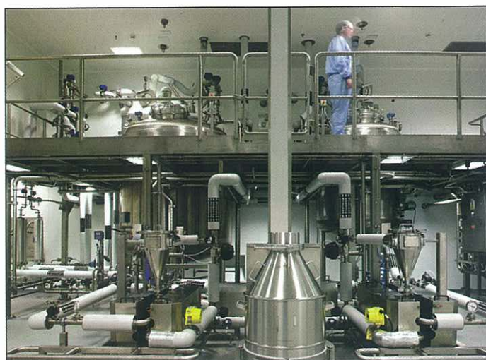
Media prep skid.
