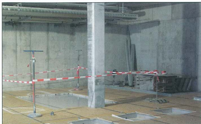
Facility mockup study. The layout details are drawn on a cover laid over top the finished epoxy floor.
