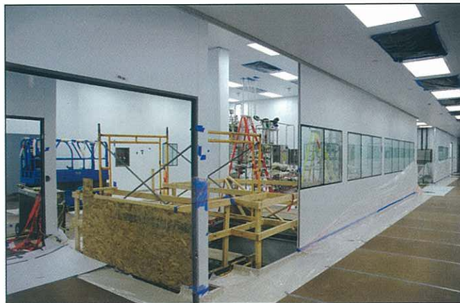
Modular cleanrooms under construction.
