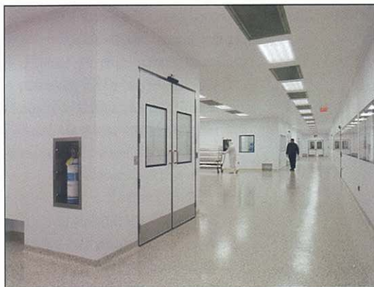
Completed cleanroom area.
