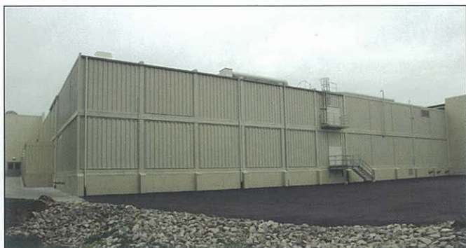
Rear view of the modular manufacturing area.
