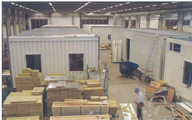
Facility modules built in a workshop environment.
